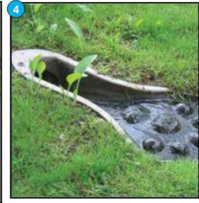
Example of Inlet Headwall w/ Energy Dissipator (Ref. 2 - Figure 28.3)
