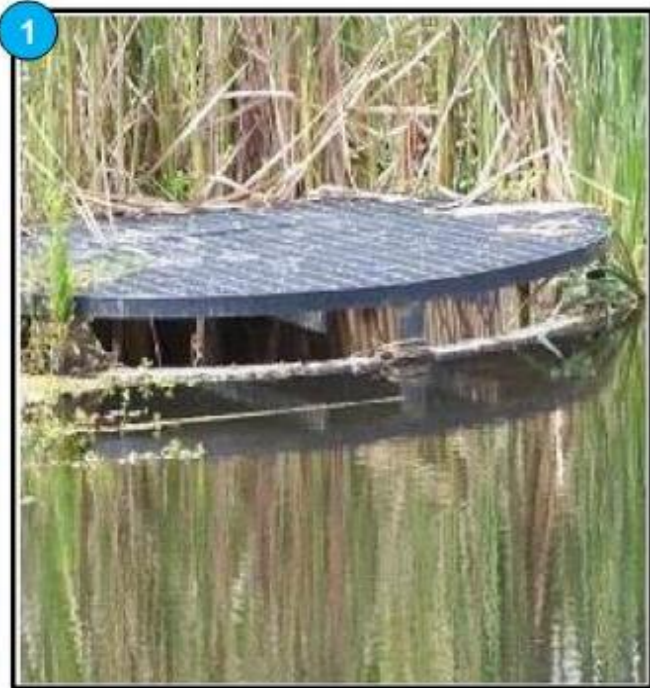
Example of Overflow Pit with Debris Screen (Ref. 1 - Figure 4.7)
