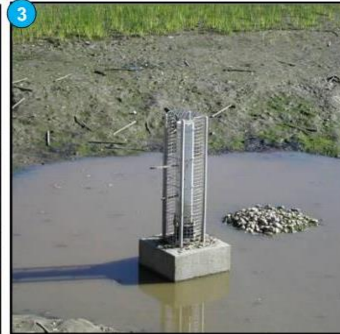
Example of Riser Outlet Pipe (Ref. 1 - Figure 10.11)
