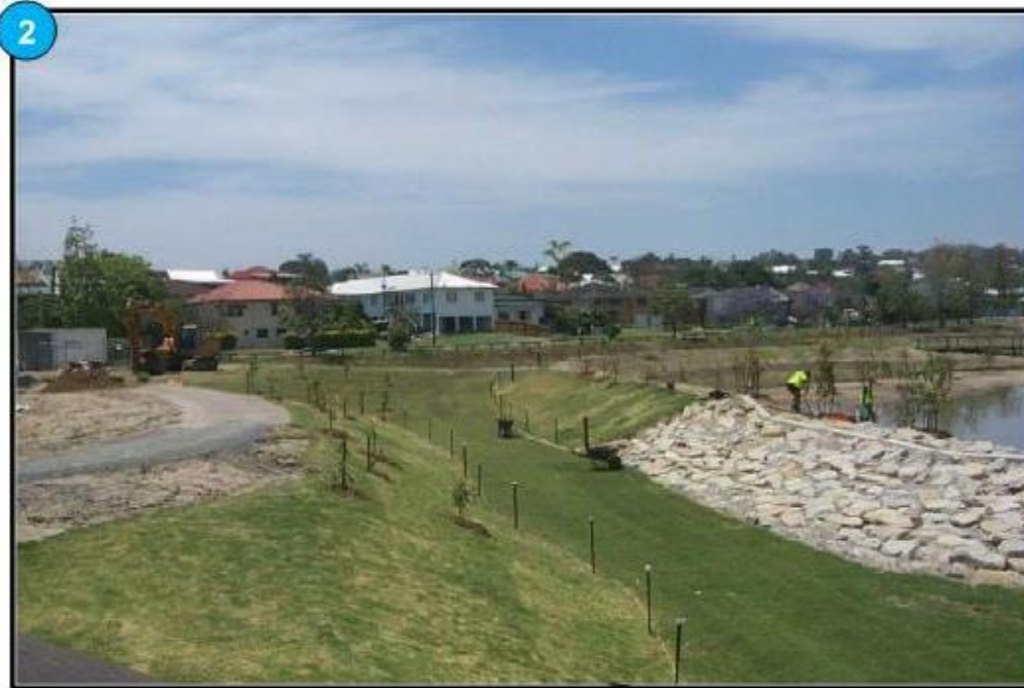
Example of High Flow Bypass Channel (Ref. 1 - Figure 10.2)
